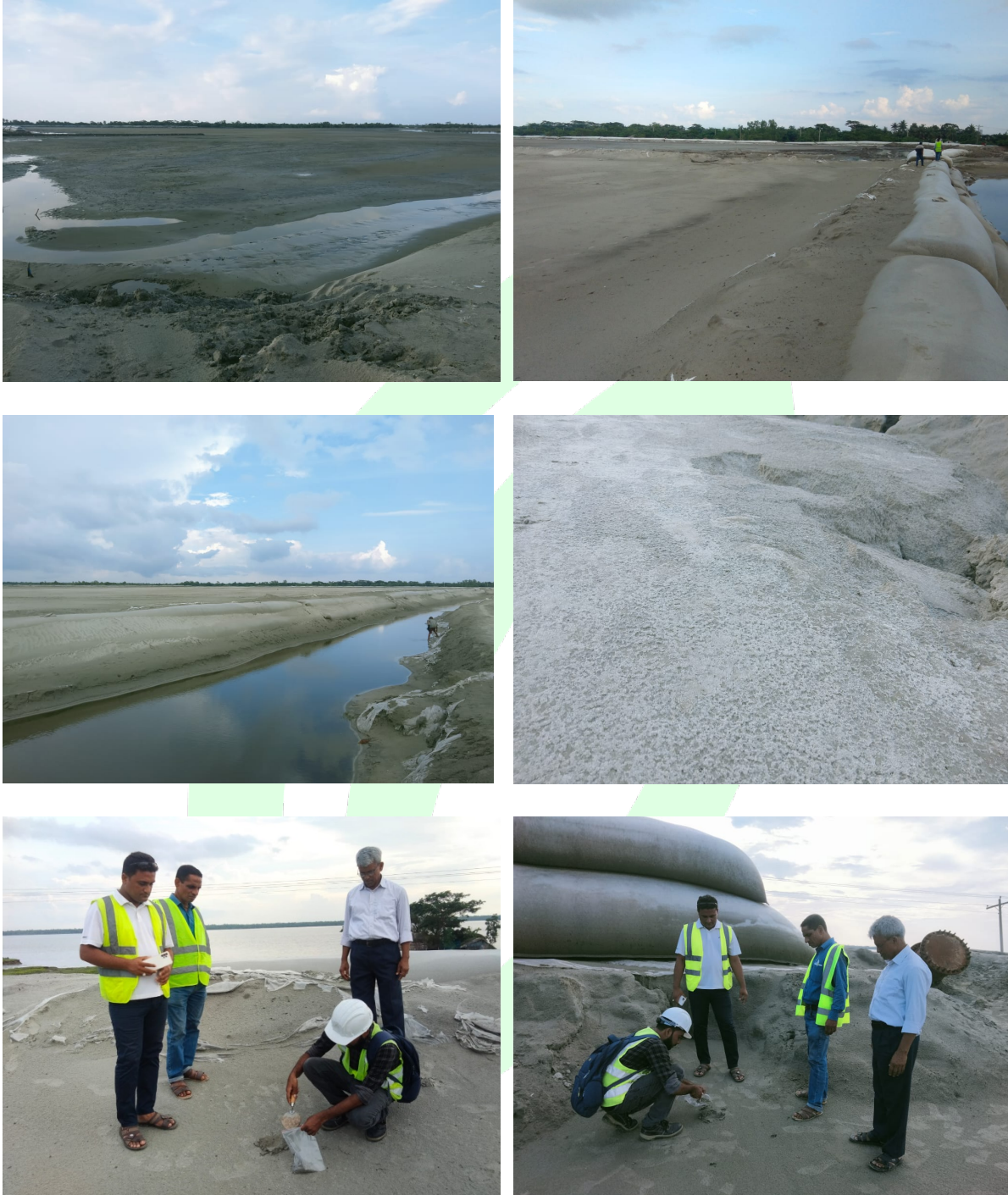
Figure: Pictorials of Site Surrounding and Soil Sampling
